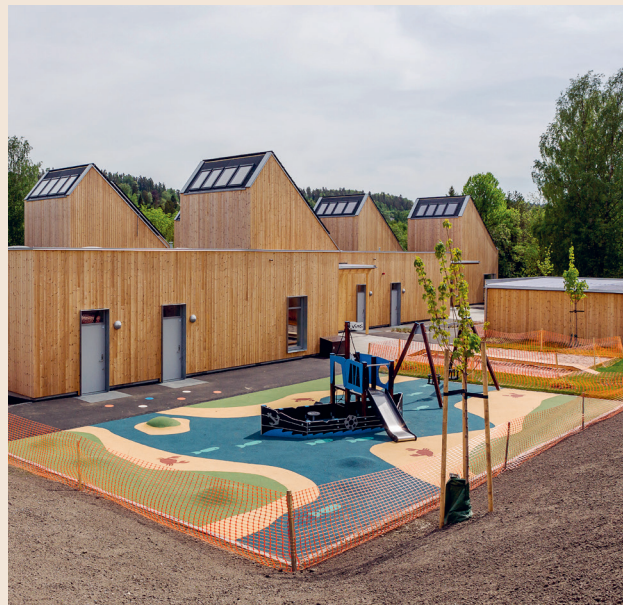
Kistefosdammen daycare centre
